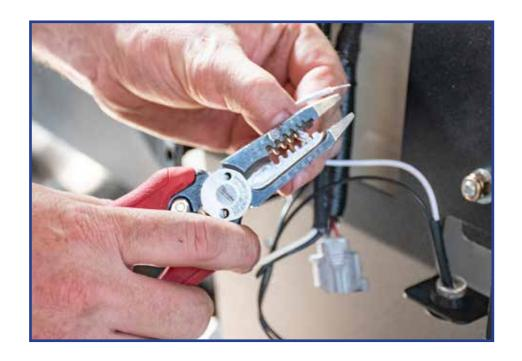
Attach the wire spades and clamp down with tool
