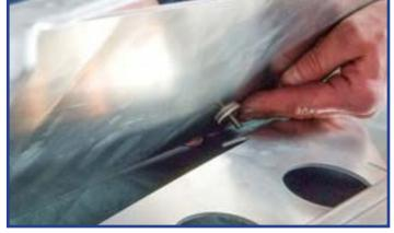
Install the weather stripping to the bottom of front fascia as shown right and trim any excess.
