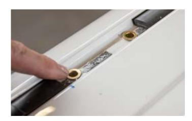
We recommend adding some sealant around the holes to provide more weather resistance from the elements as shown to the right.
